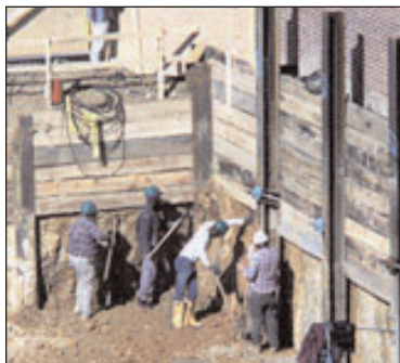
Figure 12: Installation of Soldier Pile System
